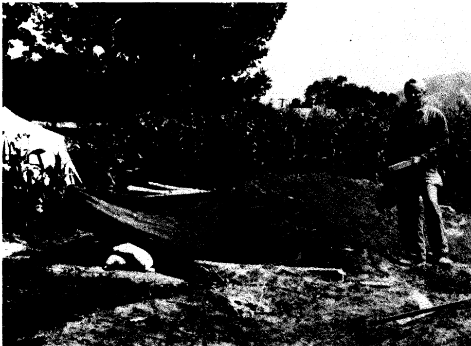
Fig. 5.6. Earth mounded over a 3\frac{1}{2} -foot-wide Pole-Covered Trench Shelter. The canvas canopy would protect the vertical entry against both fallout and rain. (A smaller canopy over the air duct-emergency exit at the other end is obscured by the mounded earth.)
