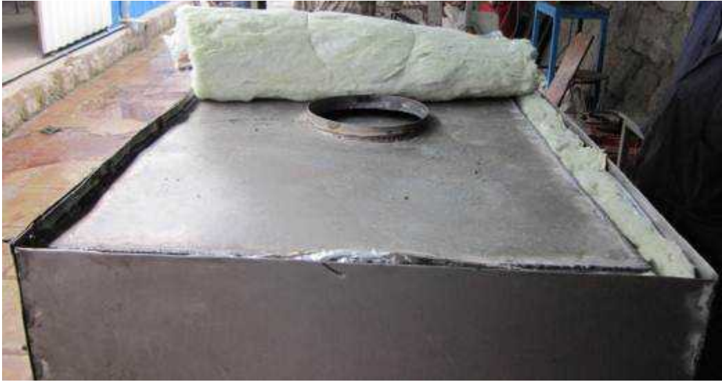
Picture 64: Image of top fiberglass piece added
