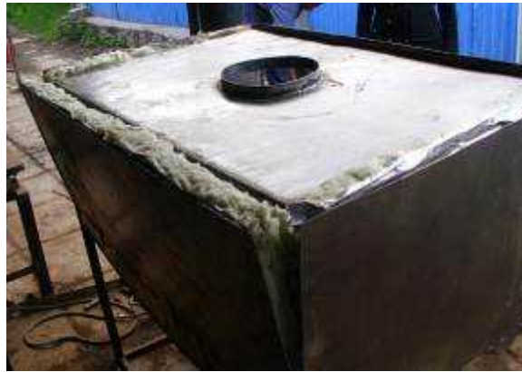
Picture 63: Image of back piece of fiberglass inserted
