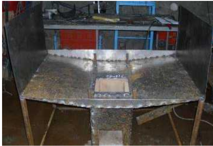
Picture 49: Image of supports attached
