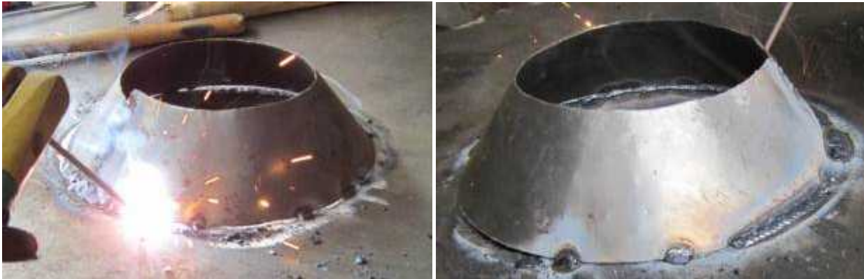
Picture 68: Images of the welding for a hermetic seal
