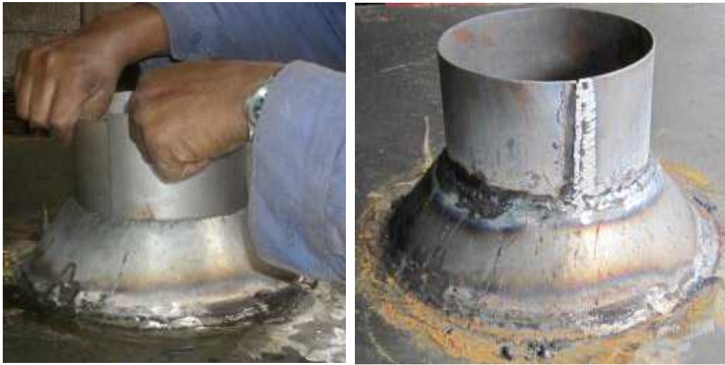
Picture 69: Images of chimney welded for a hermetic seal
