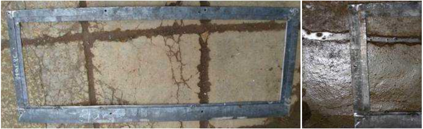
Picture 28: Top and bottom (left) and side (right) bolt holes
