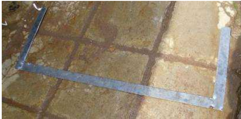
Picture 24: Image of sides welded for baking chamber flange
