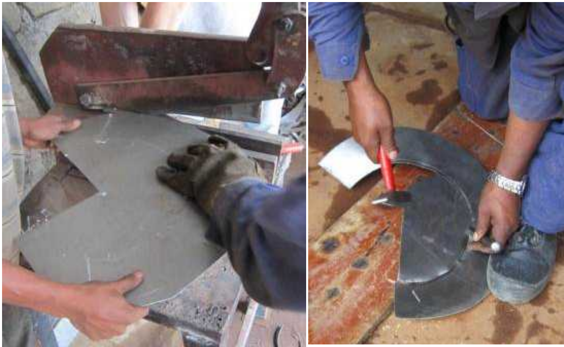
Picture 66: Images of manifold being cut
