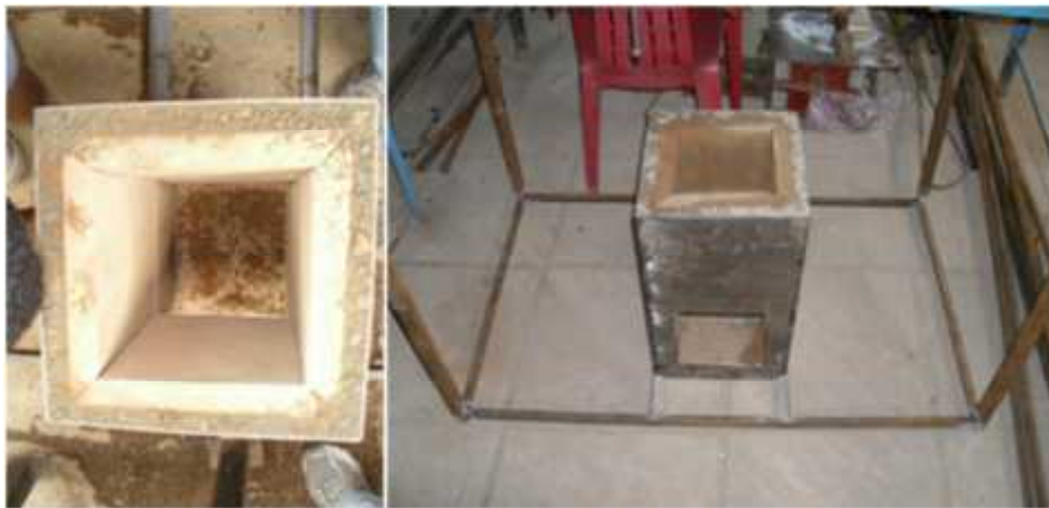
Figure 23: Addition of last tile (left) and complete combustion chamber (right)
