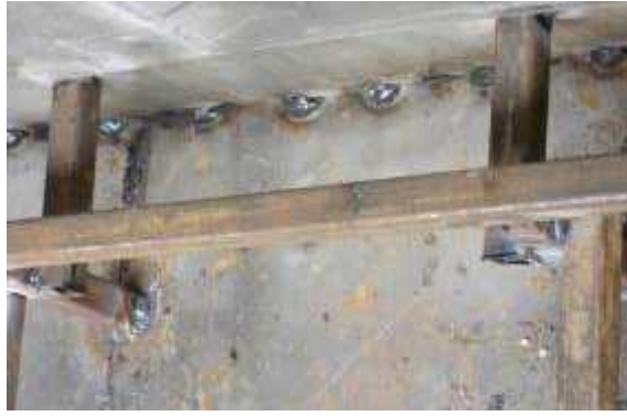
Picture 57: Close-up view of supports
