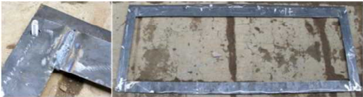
Picture 29: Magnified view of bolt through hole (left) View of all bolts attached the oven chamber flange (right)
