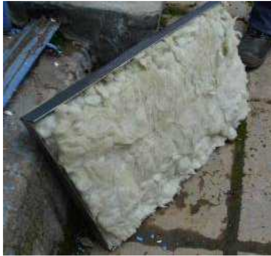
Picture 41: Image of insulation added
