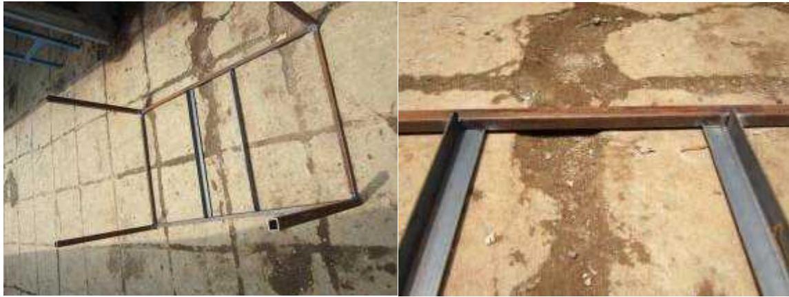
Picture 6: Image of first (left) and second (right) angle bar placement
