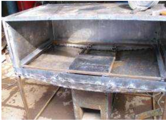
Picture 59: Image of side/top piece attached
