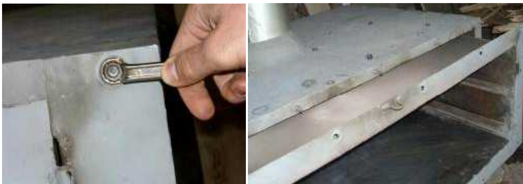
Picture 89: Image of bolt (left) and baking chamber (right) removal
