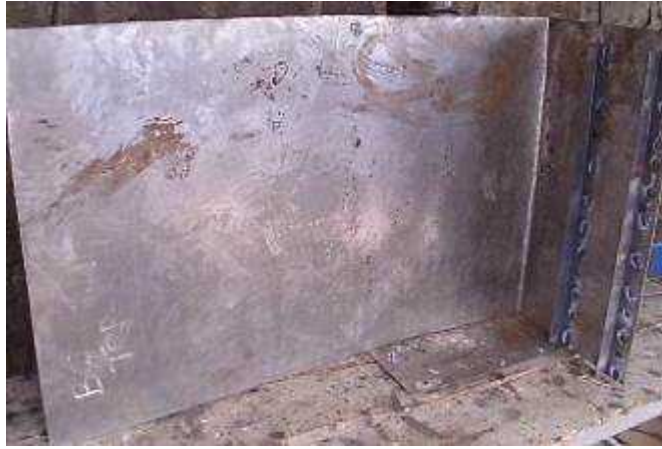
Picture 33: Image of angle bar rack supports attached
