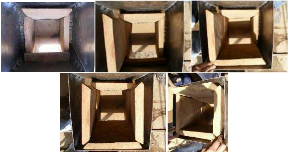
Picture 14: Placement of second layer of ceramic tiles
