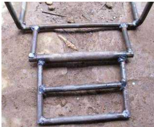
Picture 76: Image of interior bars added
