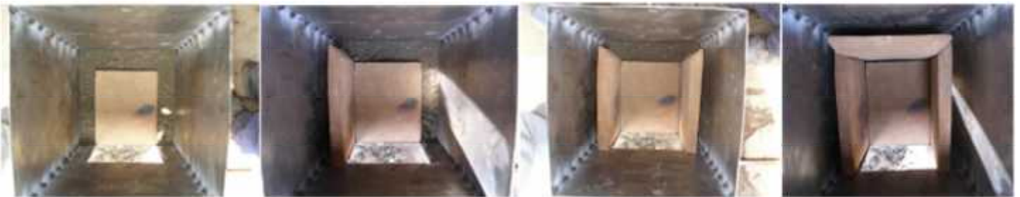
Picture 13: Placement of bottom, sides, and back tiles
